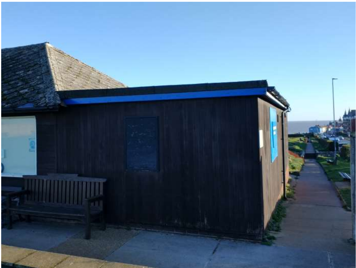
To be demolished
