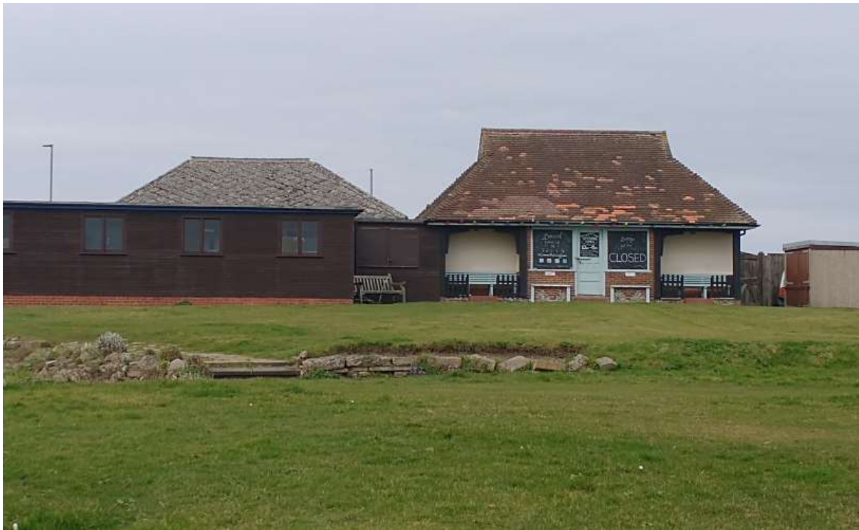
General view of the site
