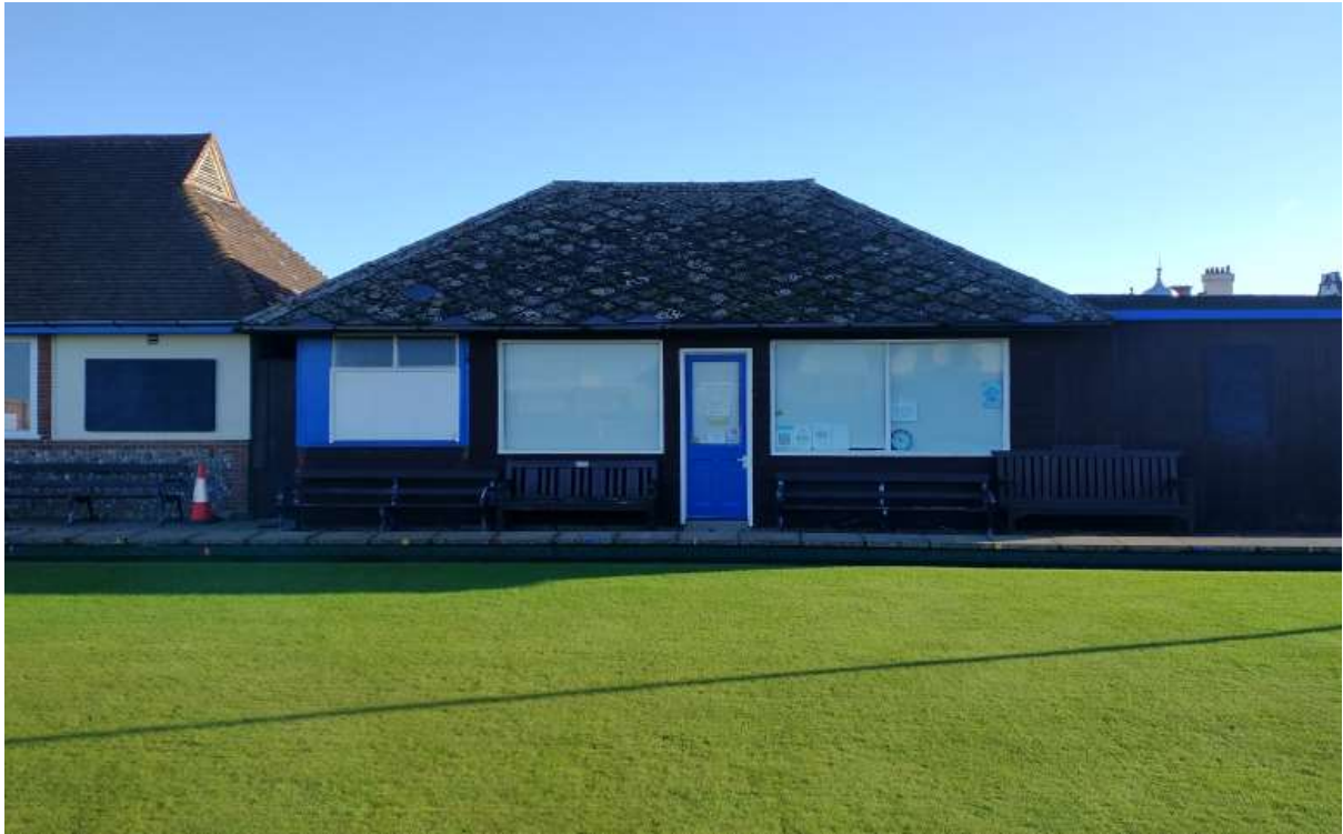
To be demolished.
